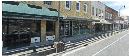
Existing Awnings will Provide Shade for Streetscape
